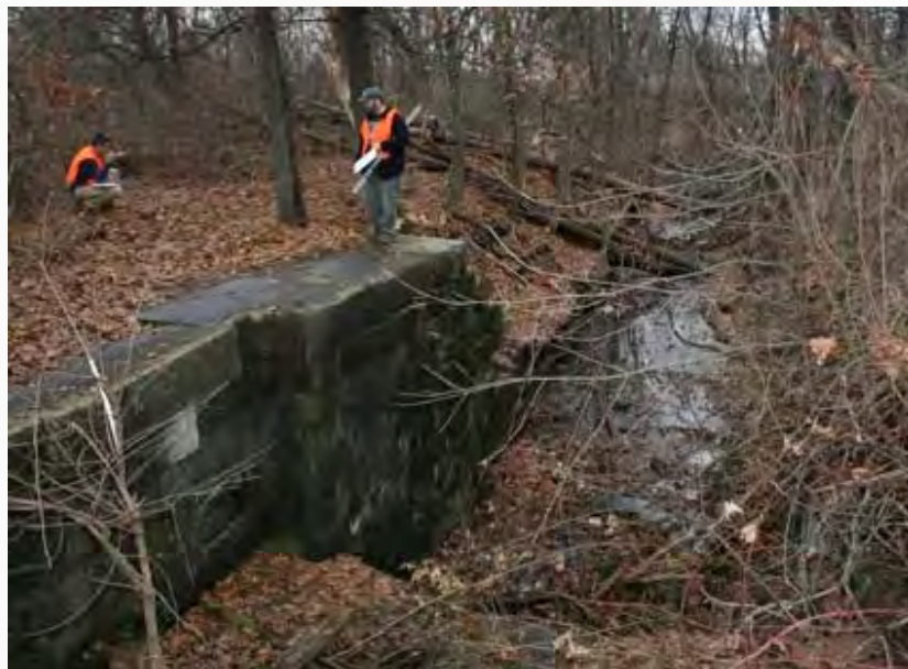
1819 Double Lock Site 42 (facing south east)
