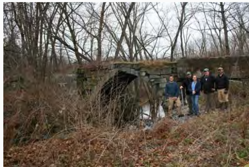
Aqueduct over Little Wood Creek with field crew Site 5A (facing north east)
